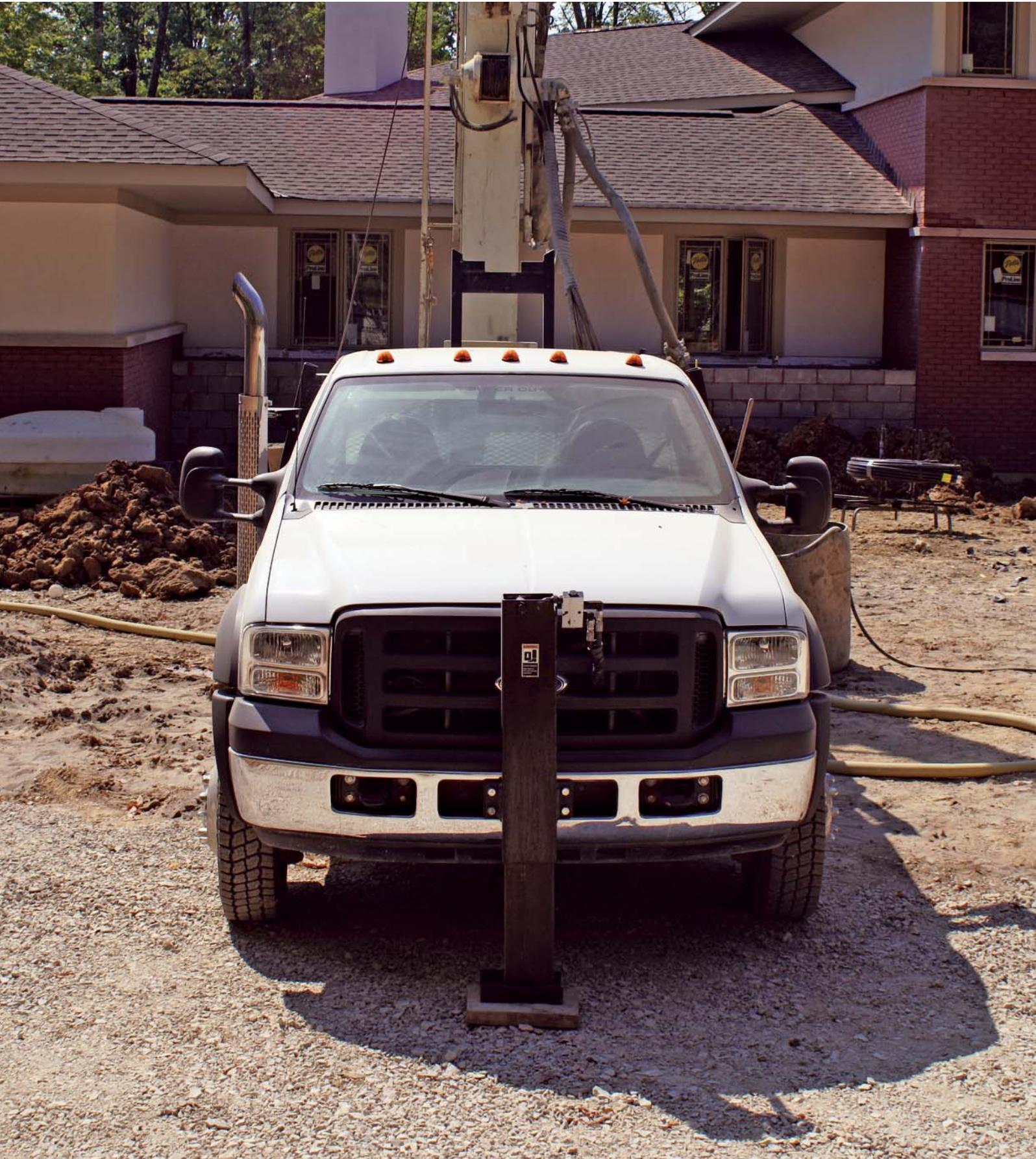
**D**ave Brennan is in a unique business — capturing the earth's energy for customers. With his company Geothermal Drilling LLC, his crews roll up to a residential home with a drill and a mini ex to install an underground loop system (a series of pipes carrying water and antifreeze) that capitalizes on the constant temperature of the earth to heat and cool homes.
